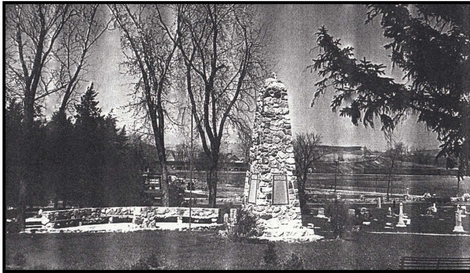
Figure 27 – Civil War Monument, amphitheater, and rostrum, 1939, looking NE.
