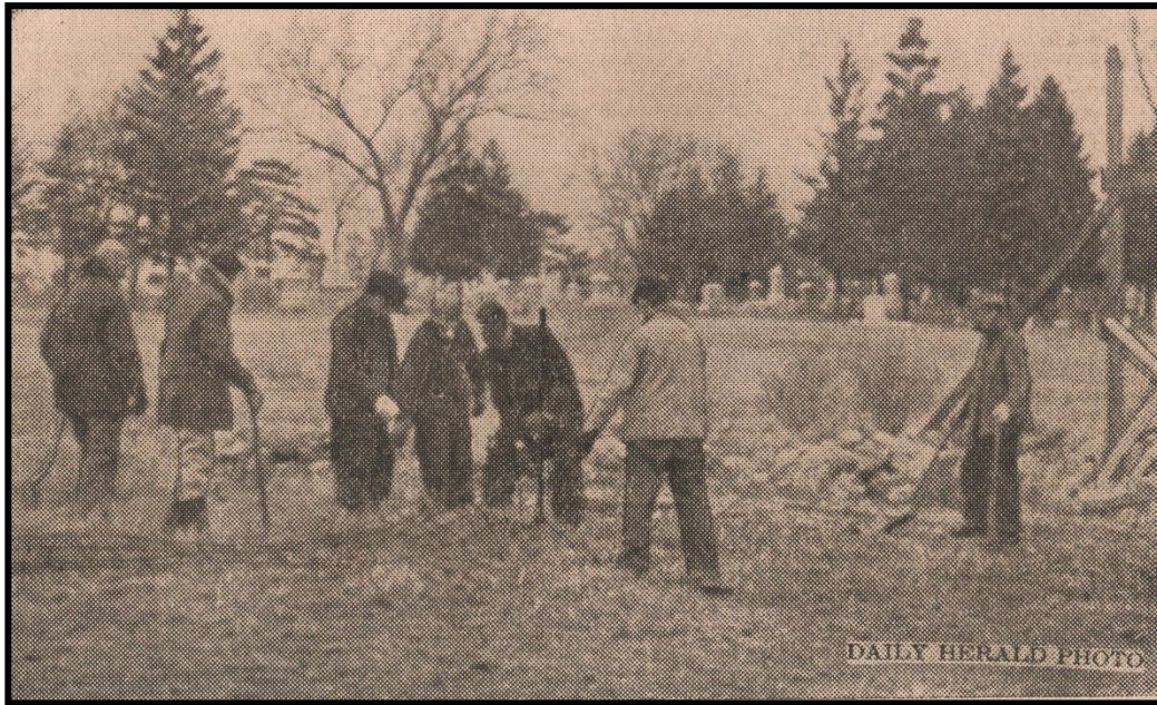
Figure 29 - WPA workers prepare the site for the east gateway looking W.
