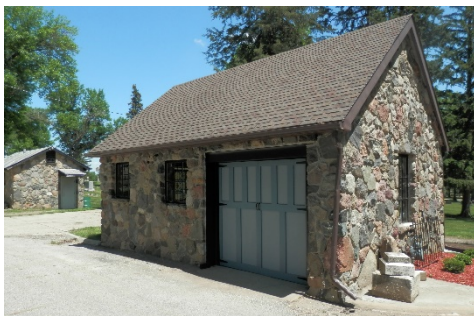
Figure 10 – Cemetery shelter house from southwest – May 25, 2018
