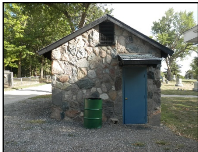
Figure 11 – Restroom building from south – Sept. 2020
