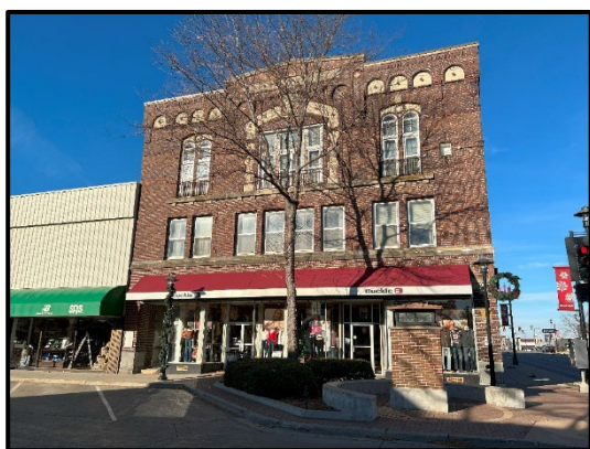
The Buckle Building
