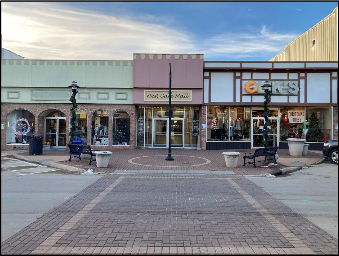
Existing Entrance from Adams Street
