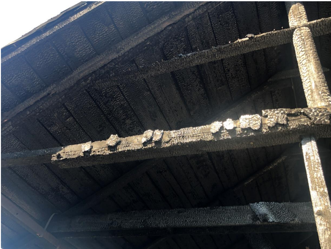
Photo 13. Roof decking and end truss framing
