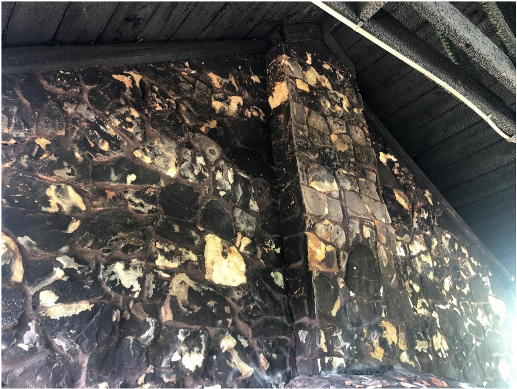
Photo 16. Fireplace rock spalling
