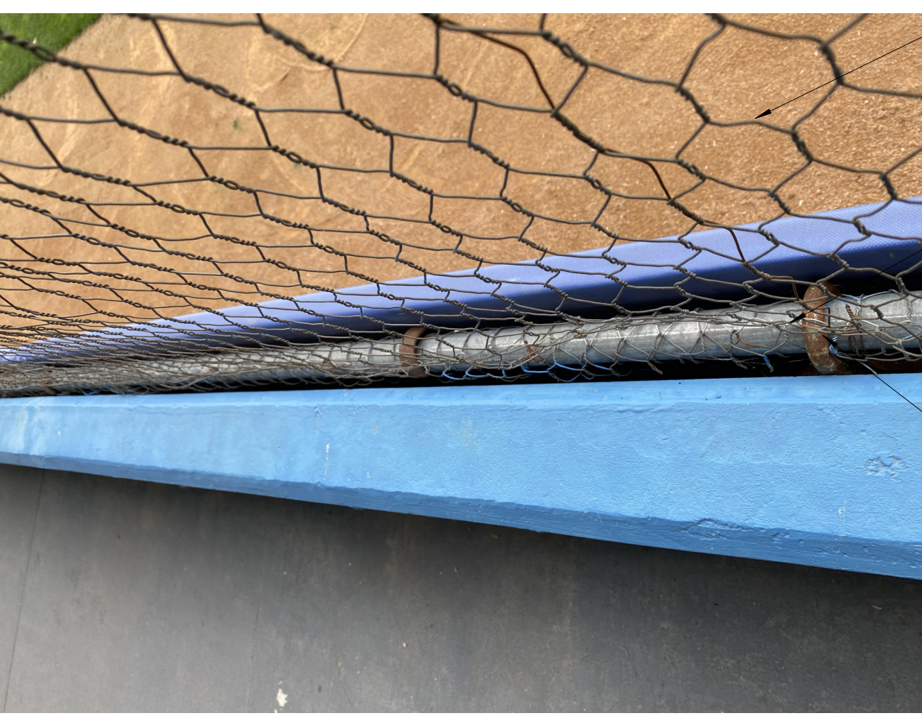
A2 SAFETY NETTING ANCHORING NOT TO SCALE
