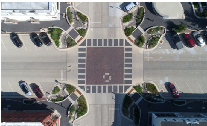
On-street angled parking is both easy to use and maximizes space in West Union.
