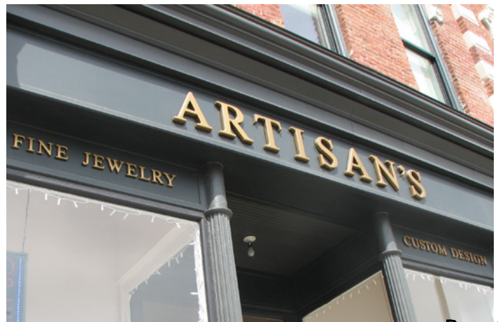
This individually mounted letter signage fits well within the storefront cornice and contributes to a traditional, elegant look.
