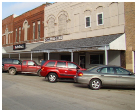
Continuous awnings fixed across multiple storefronts are inappropriate.
