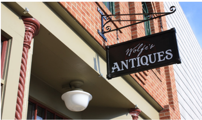
Simple projecting or blade signs are encouraged in pedestrian-oriented downtown settings and increase business visibility.
