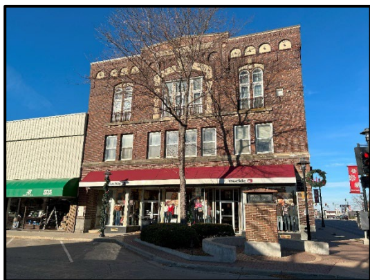
The Buckle Building
