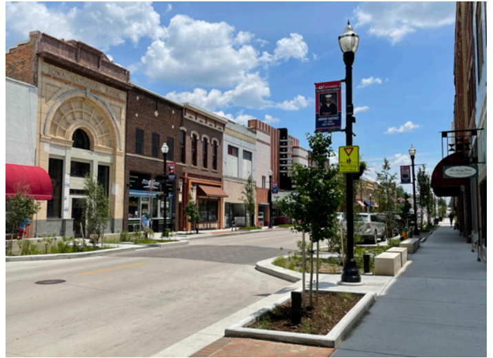
Mid-block crossings were part of a comprehensive streetscape project in downtown Ottumwa.
