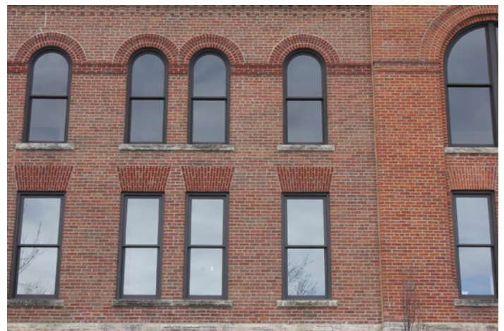
Appropriate window replacements fill the entire opening.
