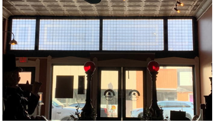
These prism glass transom windows maximize natural light and enhance the interior space.
