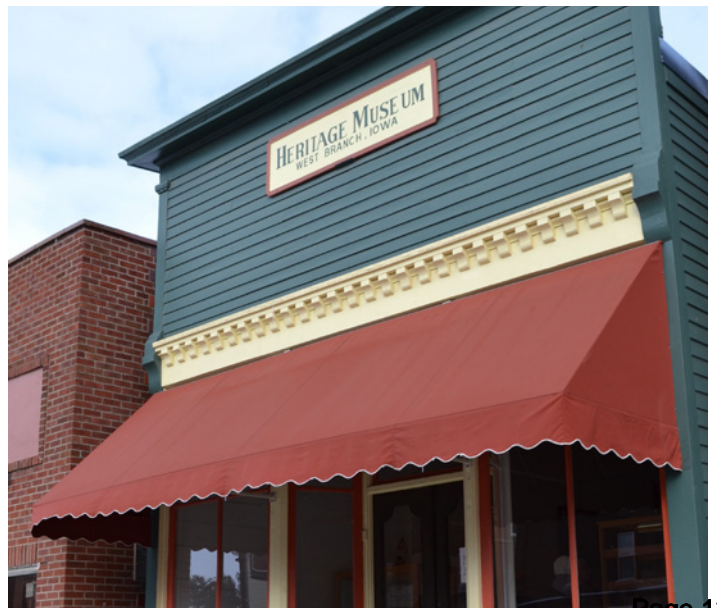
A fabric awning with a scalloped valance provides a traditional look and compliments the building's color scheme.
