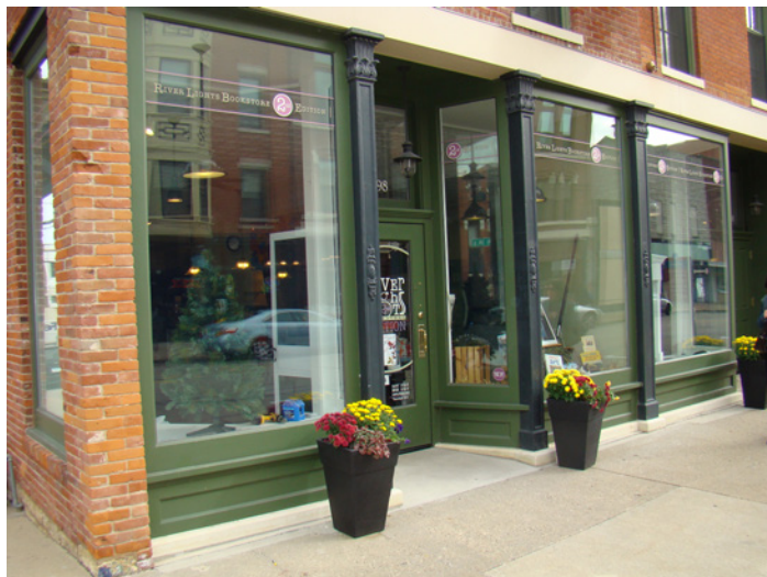
These display windows fill the full height of the original storefront opening in this reconstructed storefront.
