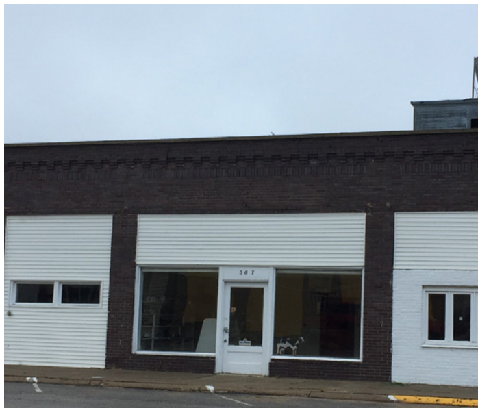
Vinyl siding creates a residential appearance and should not be used as infill or primary material on downtown buildings.
