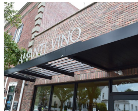
Flat metal canopies may be appropriate for specific building types.
