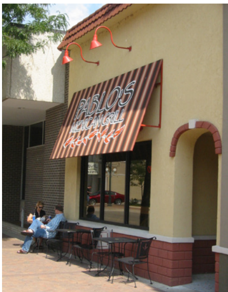
This contemporary awning fits well with the building and business.
