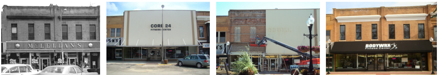
Rehabilitation of a historic building in downtown Washington included removal of an inappropriate, non-historic slipcover.
