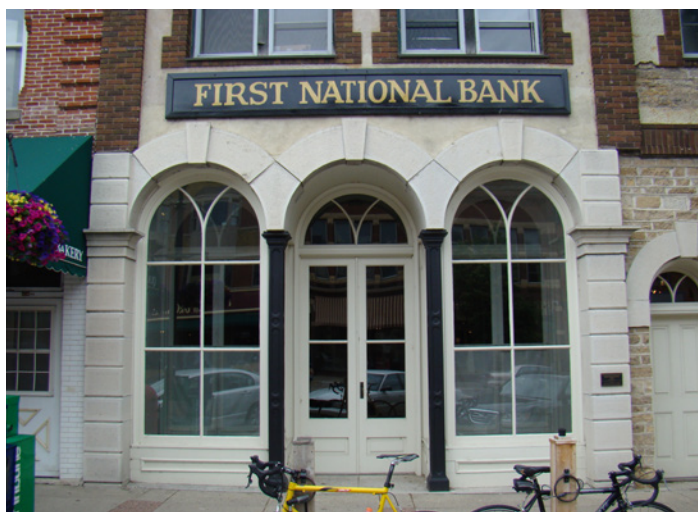
This storefront features arched openings and divided light windows, reflective of the late 1800s architecture.
