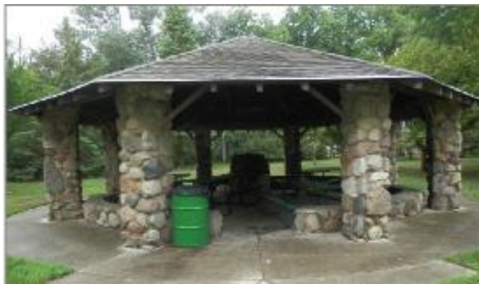
Figure 22. Open Shelter House (facing SW) June 6, 2023
