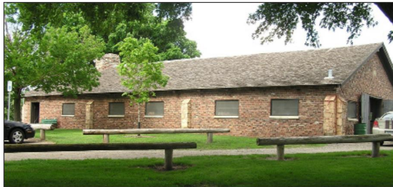
Figure 28. Enclosed Shelter House (facing NE) July 1, 2017
