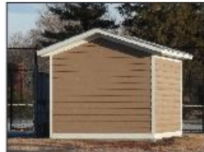
Figure 42. Tennis Equipment Shed (facing NW) Jan. 10, 2023
