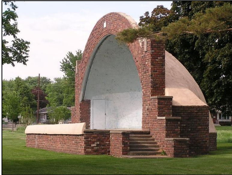
Figure 23. Band Shell (facing NE) July 1, 2017
