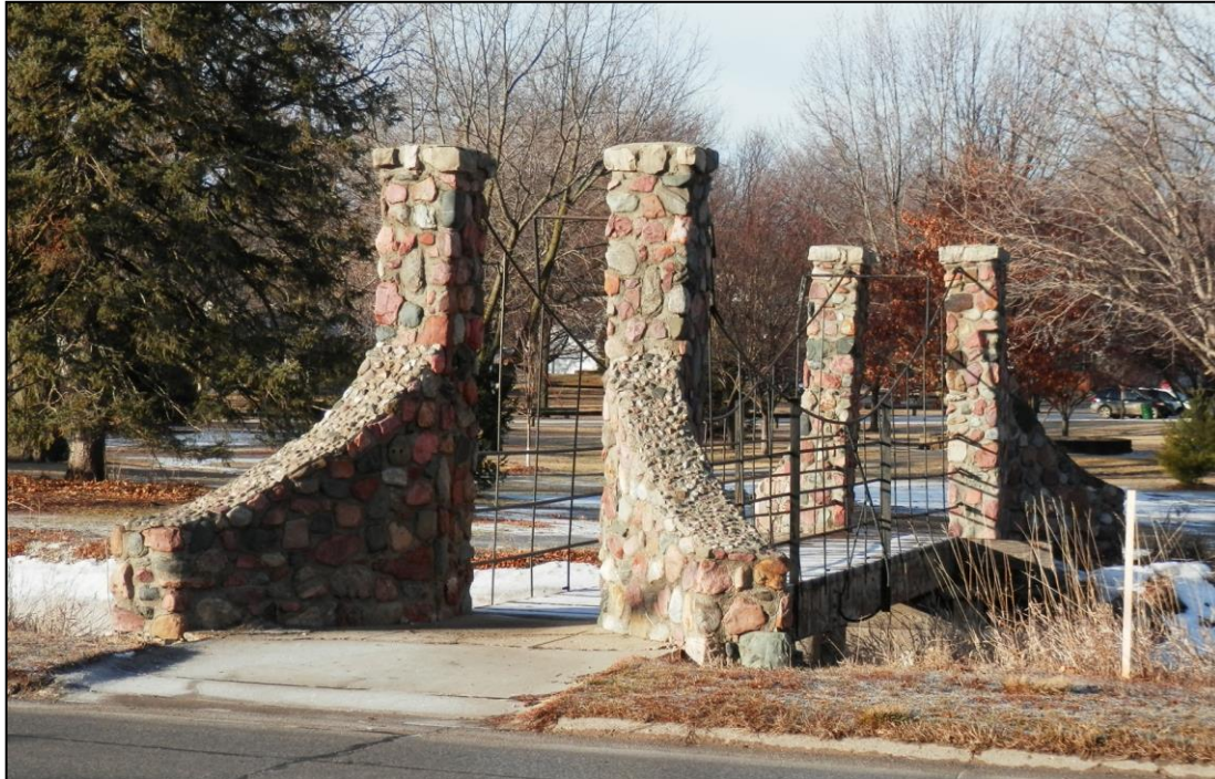
Photo 15. North Stone Footbridge (facing SW) Jan. 10, 2023
