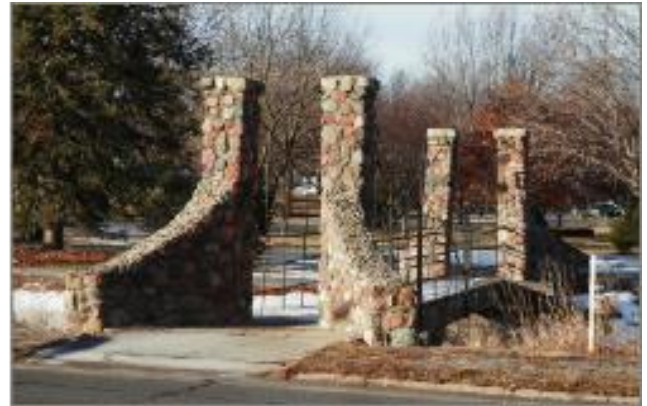
Figure 26. North Stone Footbridge (facing SW) Jan. 10, 2023
