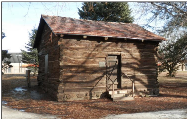
Figure 36. Trappers' Cabin (facing SE) Jan. 10, 2023
