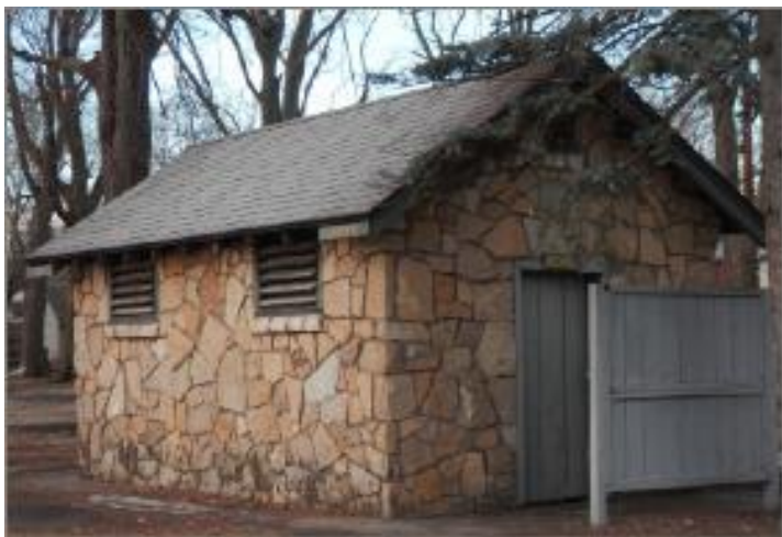
Figure 19. 1950 Restroom (facing SW) Jan. 10, 2023
