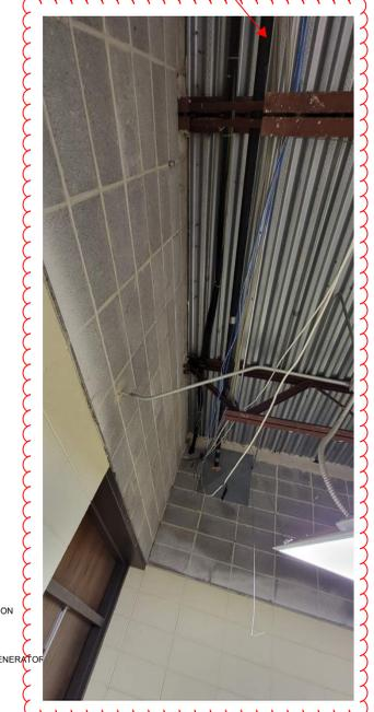
RECONNECT HARD WATER MAIN APPROXIMATELY HERE TO AVOID NEW STAIRWELL MATCH EXISTING PIPE SIZE (ESTIMATED SIZE IS 1") AND PROVIDE INSULATION
