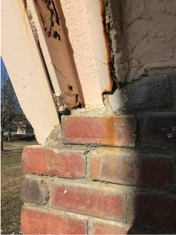
Detail of Proscenium Arch bearing on Masonry Pier – north side.
