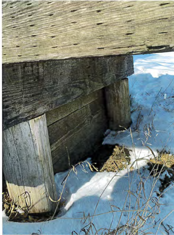
Photo 7: West abutment wall and crossbeam
