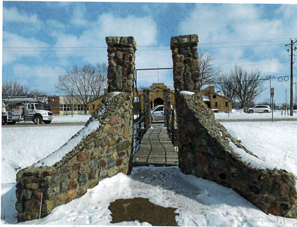
Photo 10: Leaning columns at west abutment
