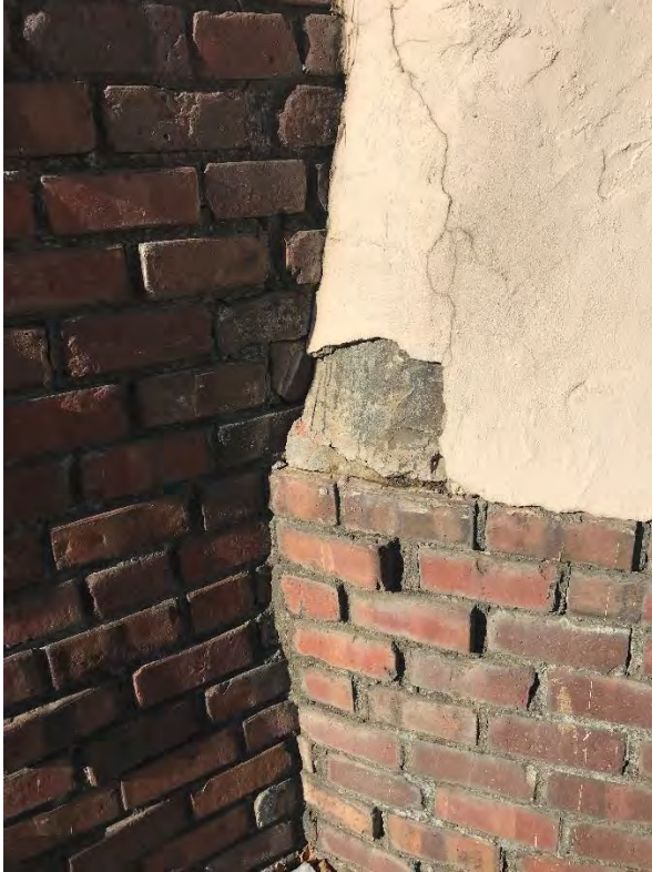
Detail of joint between dome and wall.
