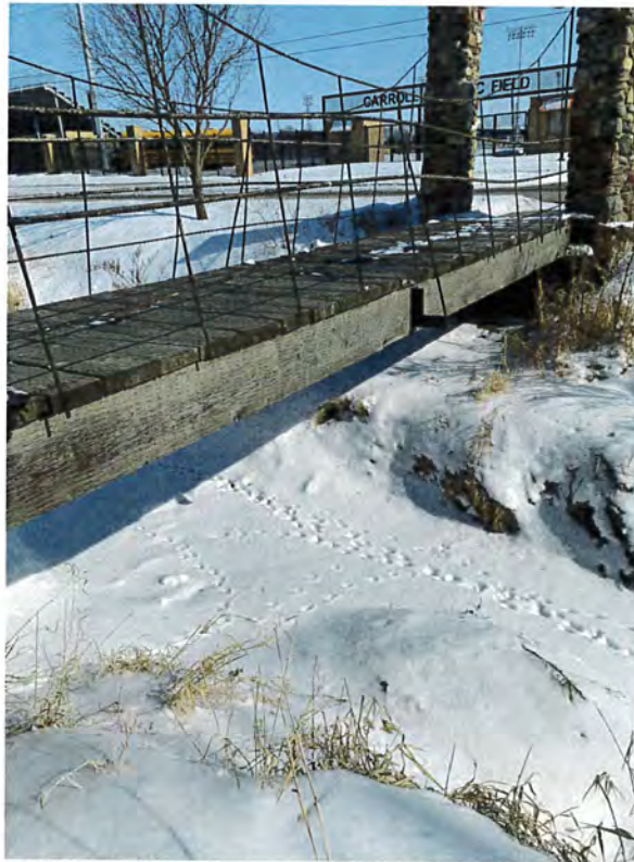
Photo 9: Slope below west abutment is about 1:1
