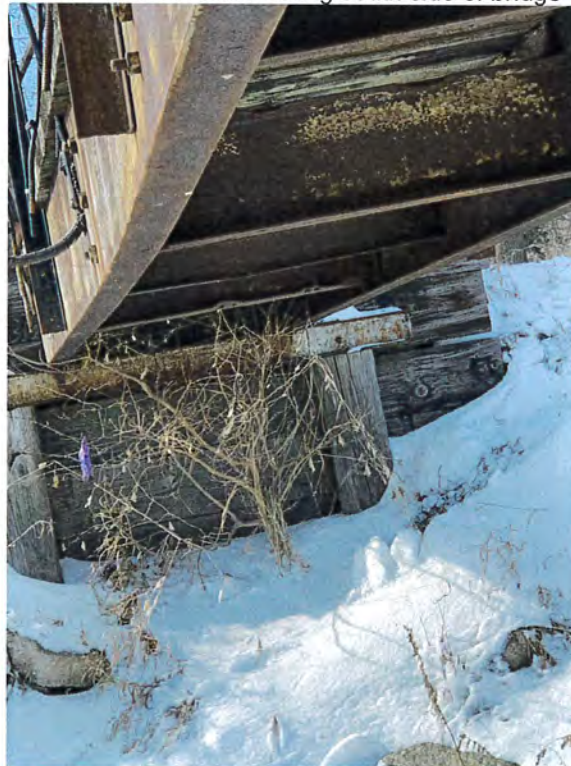
Photo 15: Crossmembers at underside of bridge
