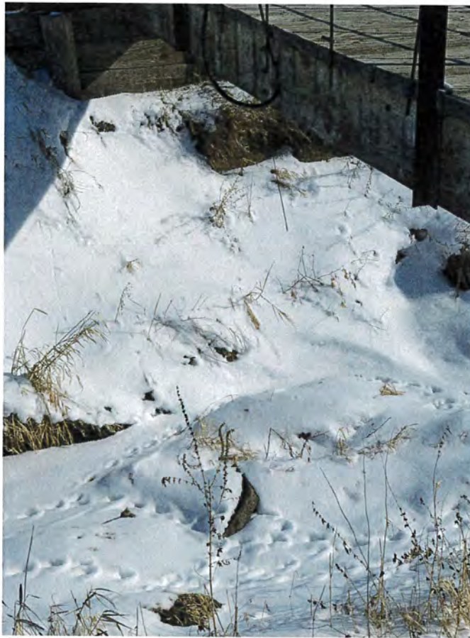
Photo 18: Slope below both abutments is steeper than 1:1
