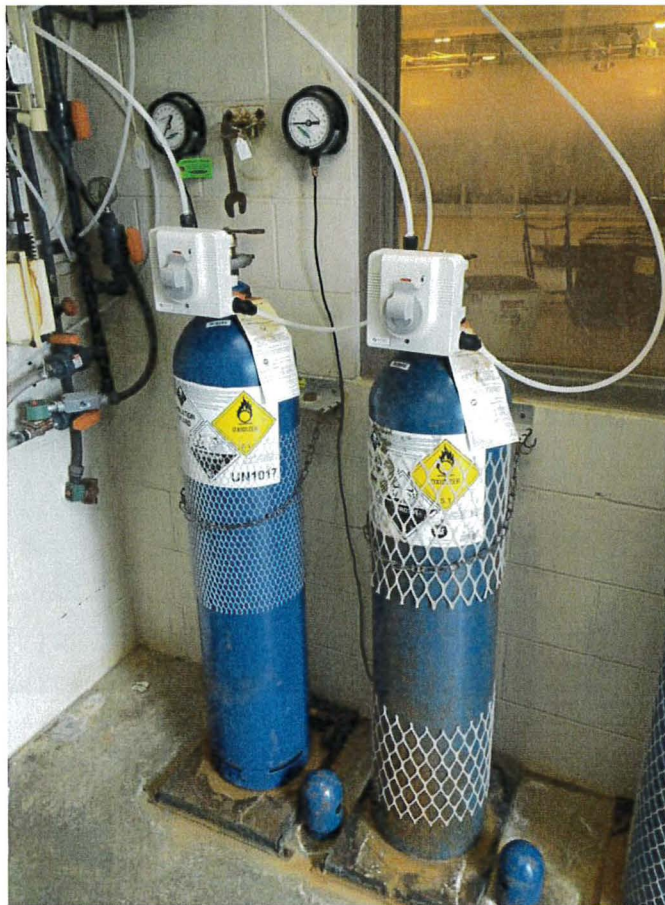
Figure 2-6: Gas Chlorine Feed System
