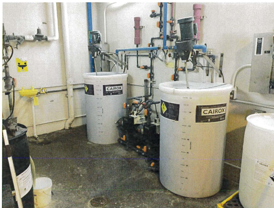
Figure 2-7: Potassium Permanganate Feed System
