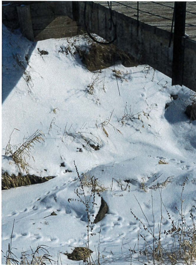
Photo 18: Slope below both abutments is steeper than 1:1
