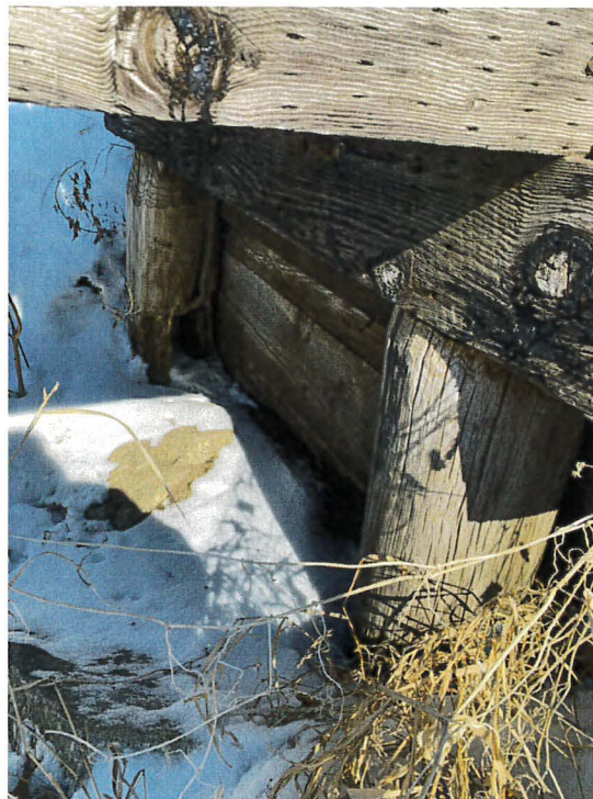
Photo 8: North wood pile hollowing out at east abutment
