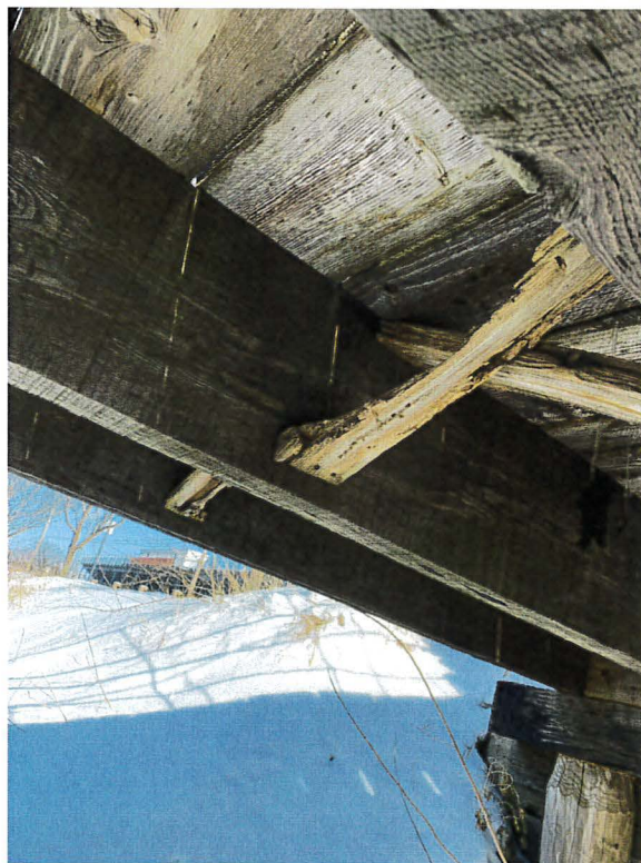
Photo 6: Beam crossmembers in poor condition near east abutment
