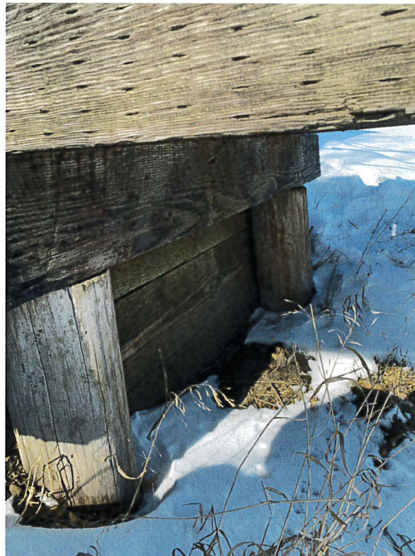
Photo 7: West abutment wall and crossbeam
