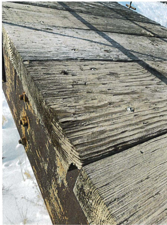
Photo 12: Walking surface plank showing some wear and tear
