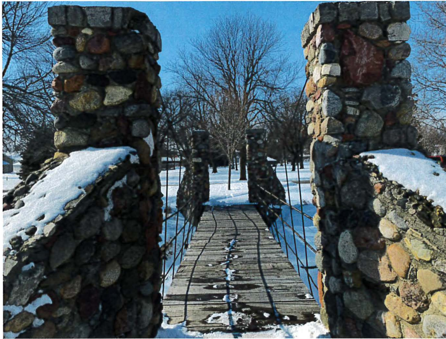
Photo 1: Looking west from east abutment, leaning column near side on right
