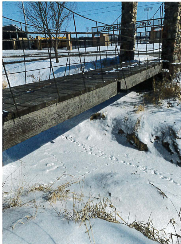
Photo 9: Slope below west abutment is about 1:1
