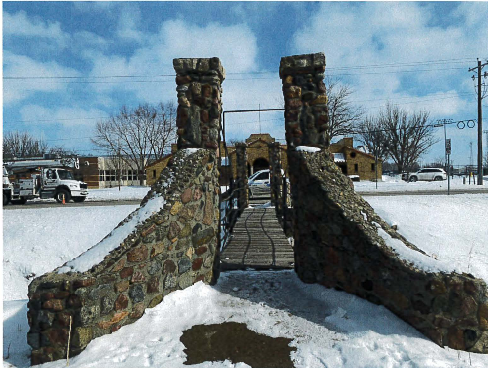
Photo 10: Leaning columns at west abutment
