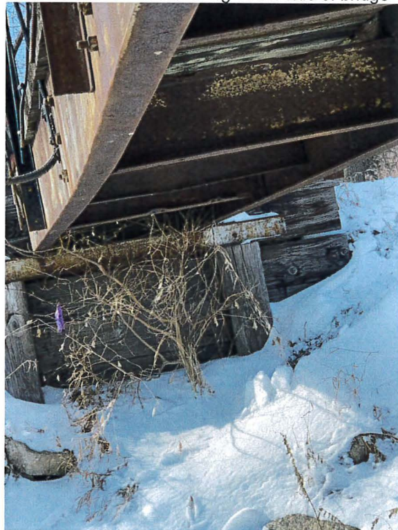
Photo 15: Crossmembers at underside of bridge
