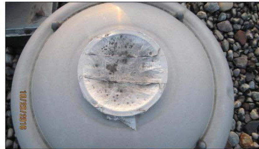
Figure 24: Duct tape has been installed over a missing cap on one of the exhaust fans. Figure 25 shows a properly installed cap.
