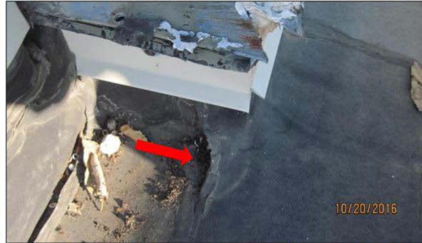
Figure 15: South east elevation – the EPDM joint has separated and the base of the precast wall, area shown with red arrow.
