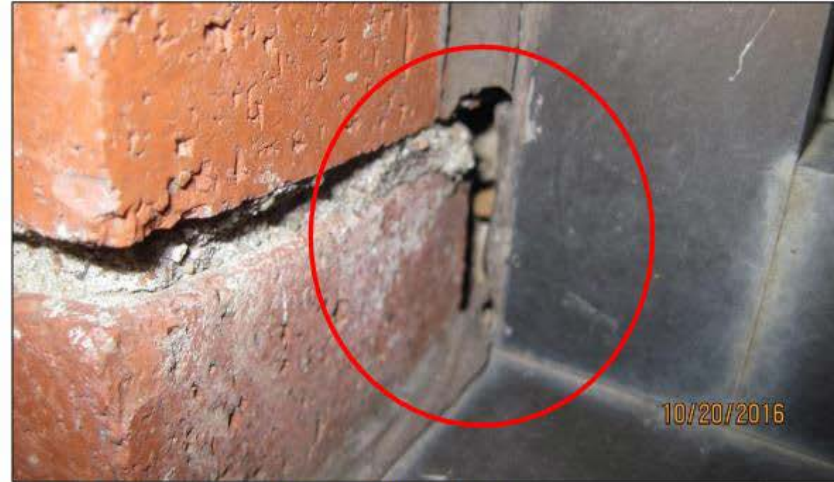
Figure 7: Additional failed window to masonry joint, area outlined in red
