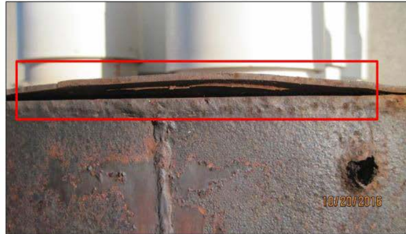
Figure 20: The cap on the large stack is separating, area outlined in red.
