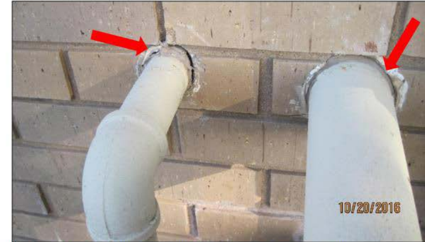
Figure 17: South elevation - two mechanical penetration are no longer permanently sealed.
