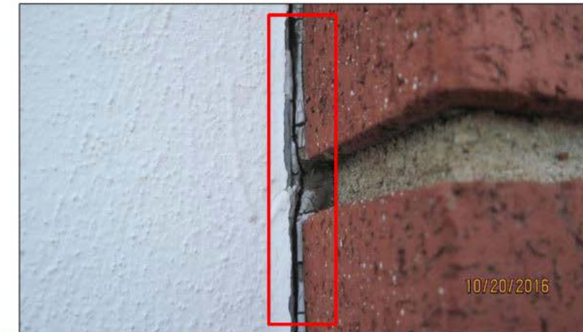
Figure 14: Failed plaster to masonry control joint, area outlined in red.
