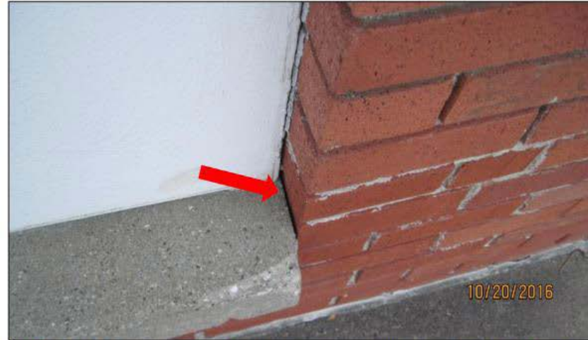
Figure 15: The sill at the base of plaster is not sealed at the masonry connection, area show with red arrow.
