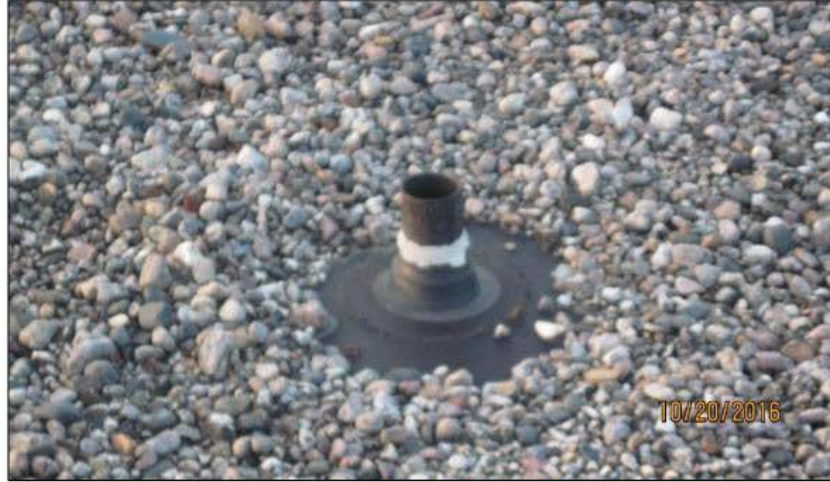
Figure 27: It appears one of the roof boots on the south flat roof has been repaired. This installed secondary sealant does not appear to be an EPDM product.
