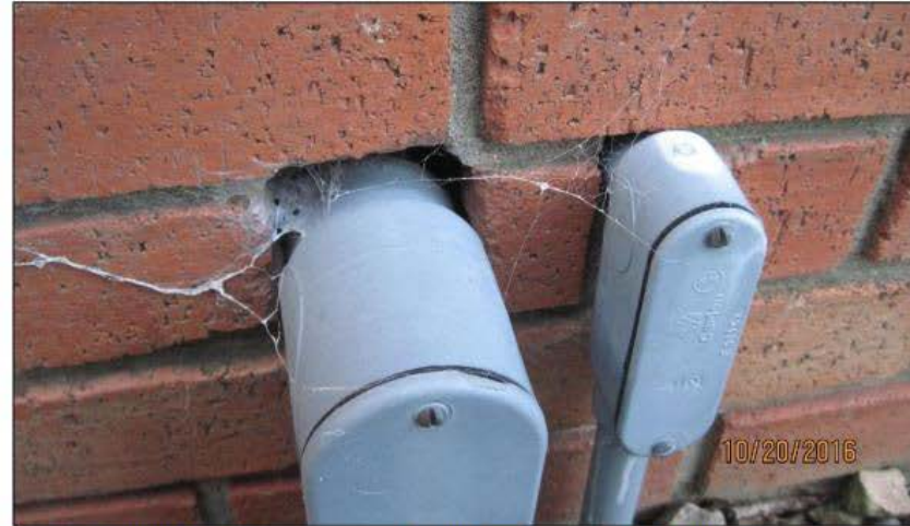
Figure 19: The electrical conduits on the north elevation are not completely sealed at the masonry connection.
