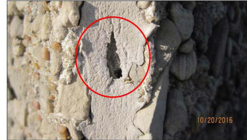
Figure 5: Failed vertical precast joint, area outlined in red.
