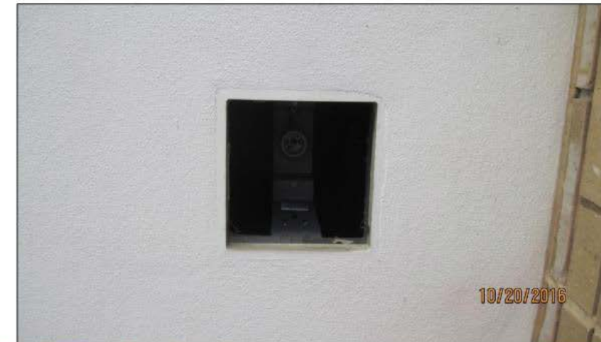
Figure 14: Missing soffit light on the north elevation.
