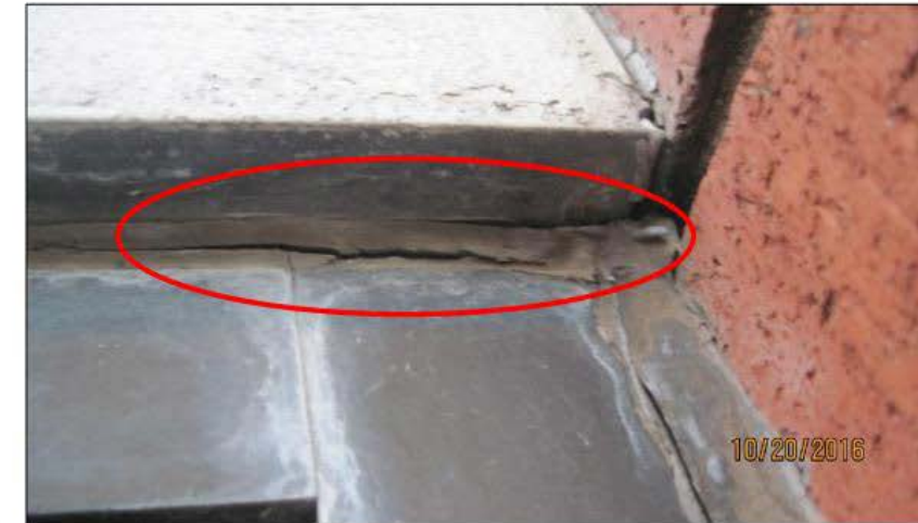
Figure 6: Failed window to lintel joint, area outlined in red.
