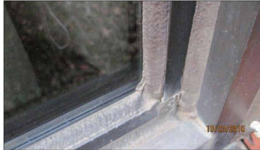
Figure 11: Some of the glazing unit's gasket connections, at the pressure plat, have been sealed with a secondary sealant.
