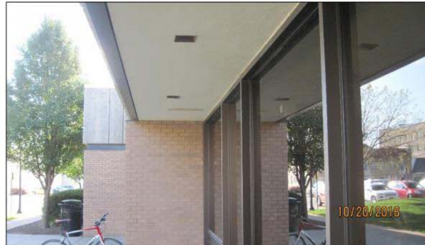
Figure 12: The soffit along the north elevation appears to be vented.
