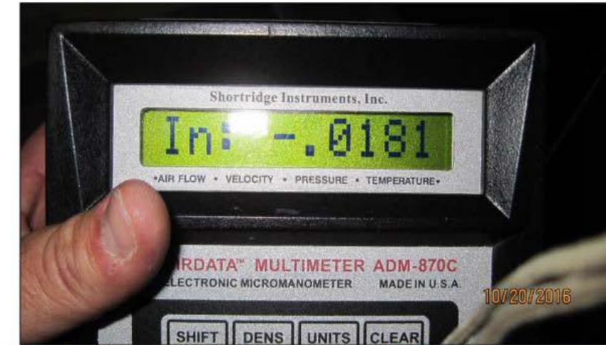
Figure 25: The building is currently operating under a negative pressure of -.0181 inches of water column.
