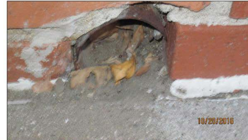
Figure 18: There is an open pipe that looks to be abandoned next to the night drop box on the west elevation.
