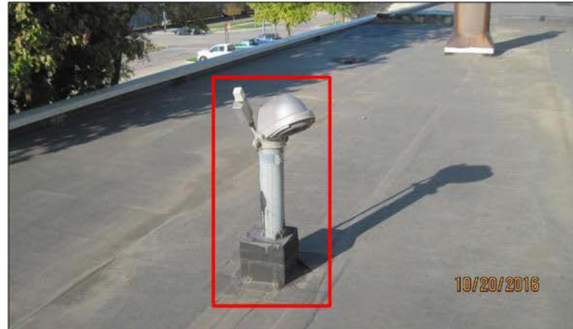
Figure 16: It doesn't appear the outlined electrical conduit is being utilized.
