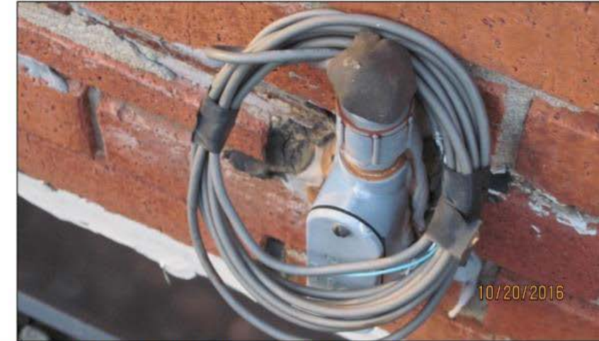
Figure 21: Same elevation as Figure 20, additional penetration that is not completely sealed.
