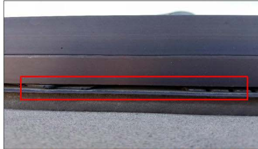
Figure 11: Additional image of the large gap between the window frame and sill flashing, area outlined in red.
