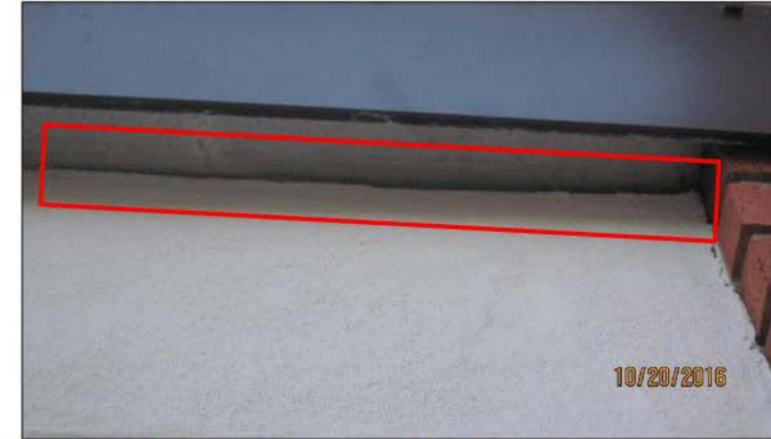
Figure 17: The plaster is not sealed to the steel lintel, area outlined in red.
