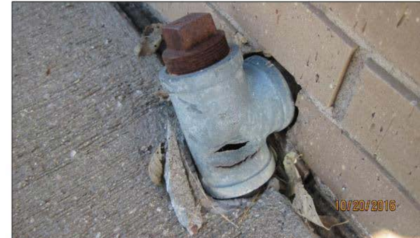
Figure 18: South elevation - additional penetration that is no longer permanently sealed.
