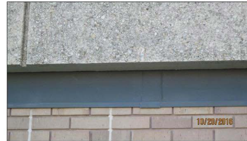
Figure 22: Sheet metal flashing is installed on to top of the masonry wall around the majority of the building.
