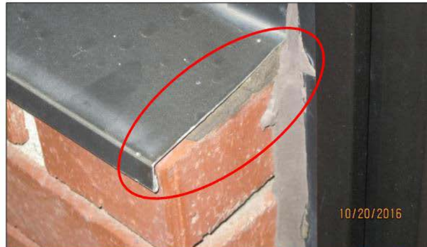
Figure 12: Masonry endcap not installed, area outlined in red. See area outlined in yellow in Figure 13 for properly installed endcap reference.
