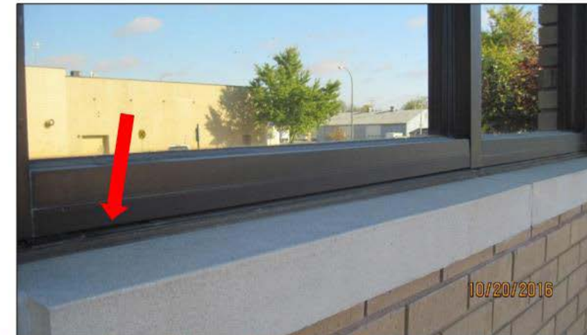
Figure 10: There are large gaps between the bottom of the window frame and the sill, area shown with red arrow.
