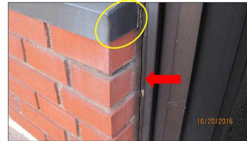
Figure 13: Failed masonry to door frame joint, area show with red arrow.
