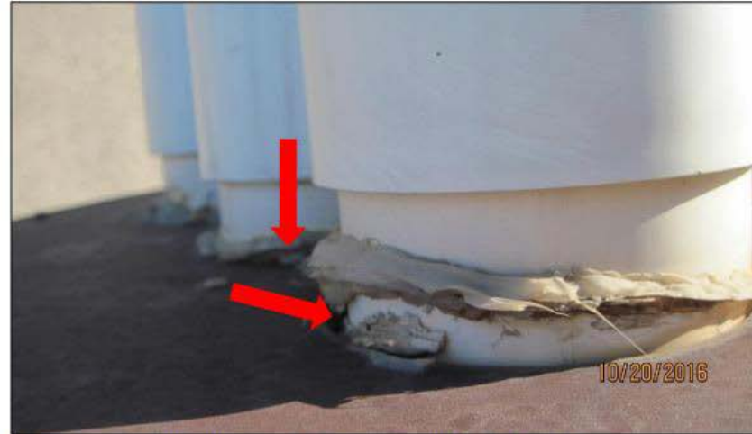
Figure 19: The PVC vent pipes are not permanently sealed, area shown with red arrows.
