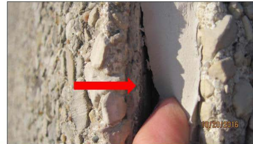
Figure 6: Additional image of a failed vertical precast joint, area shown with red arrow.
