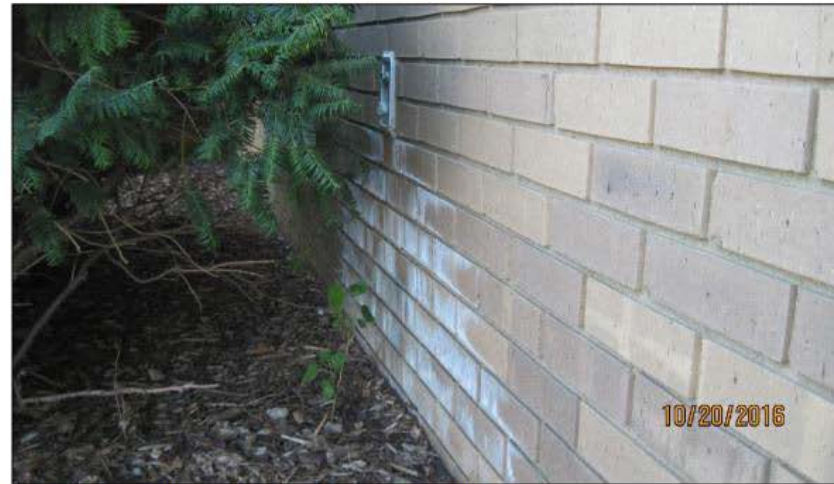
Figure 23: Efflorescence is present around a sill cock on the north elevation.
