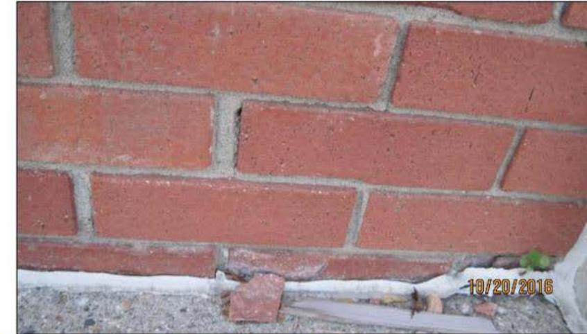
Figure 9: There are multiple areas where the masonry bricks are spalling. The control joints between the masonry walls and concrete slabs has failed.
