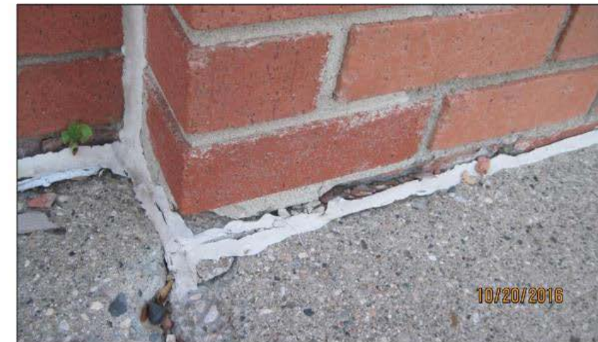
Figure 10: Additional image of spalling masonry bricks.
