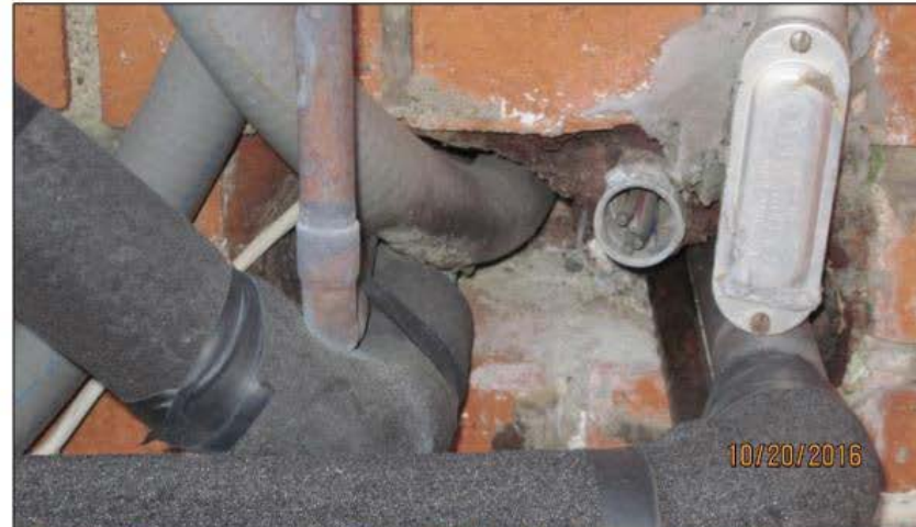
Figure 20: The north side of the upper masonry wall has multiple mechanical penetrations that are not sealed.
