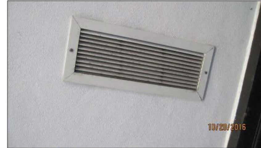
Figure 13: This appears to be a soffit vent along the north elevation.
