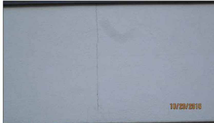
Figure 16: The plaster has a large crack on the west side of the entry along the east elevation.
